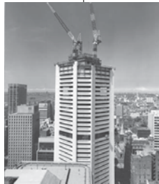
MLC Centre 1977 (228 Metres) (National Archives)
